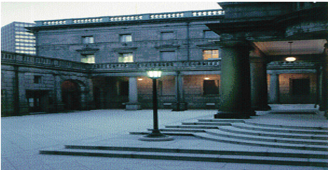
View of the BOJ courtyard around sunset
